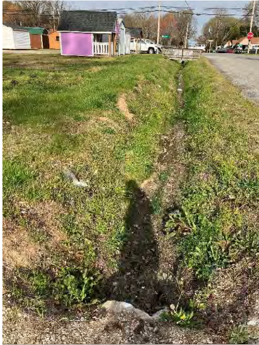
Photo 1: North side of Kansas Ave looking east
