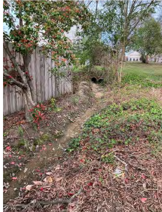
Photo 4: Looking east behind 505 Cook Street – Double barrel outlet into ditch
