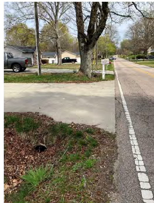
Photo 4: Looking east on Brantley - Pipe under driveway at 1307 Brantley Road
