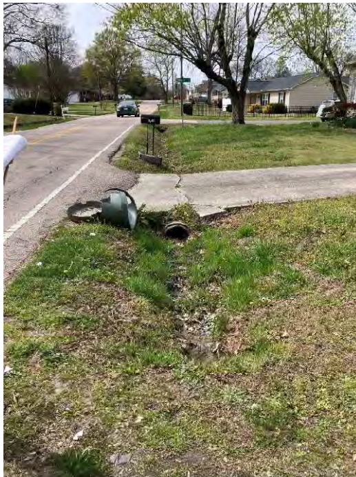
Photo 3: Looking west on north side of Brantley Road - Pipe under driveway at 1401 Brantley Road
