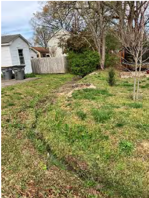
Photo 3: East side of Charles Street looking east – Ditch behind 505 Cook Street
