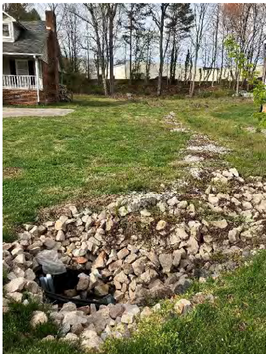
Photo 5: Rock lined channel adjacent to 618 Breckenridge Road
