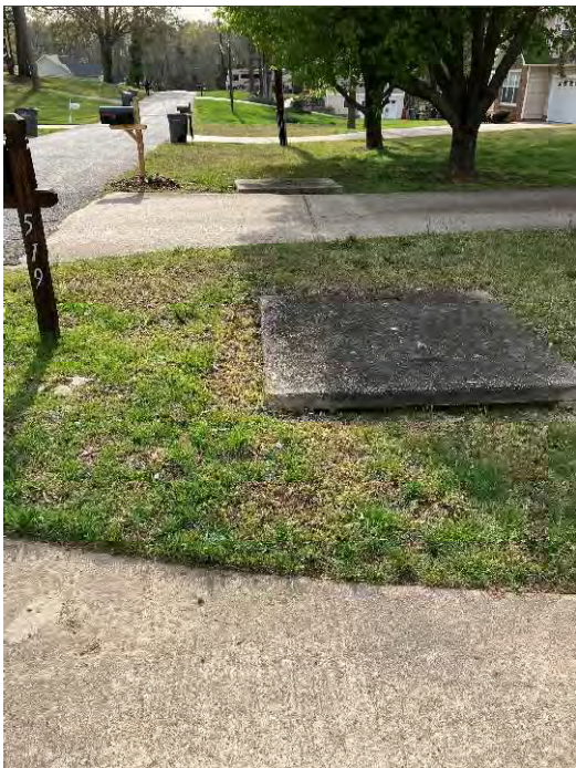
Photo 3: Slaptop inlets on north side of Kansas Street looking west
