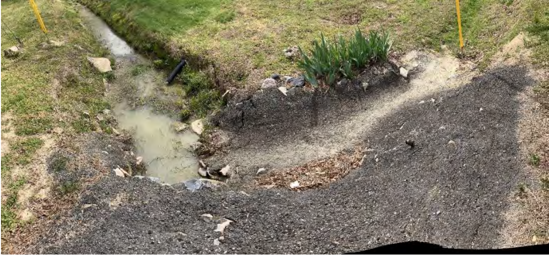
Photo 9: South side of Brantley Road looking south – Downstream outlet from Marie Avenue stormwater system
