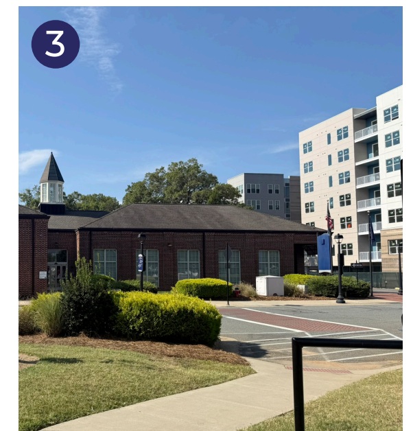
TRAIN STATION WITH "FLOATING" MID-BLOCK CROSSWALK
